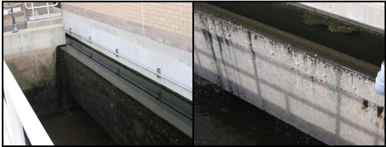
Filter Influent Weir After Cleaning
